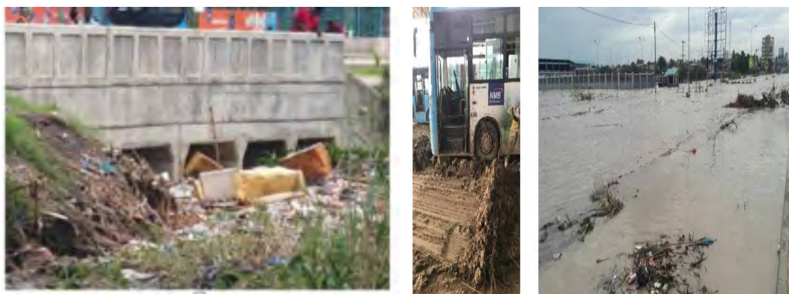
Plate 11-4: waste trapped in bridges and flooding impact at Jangwani area in Dar es Salaam City Source: World Bank (2022)
