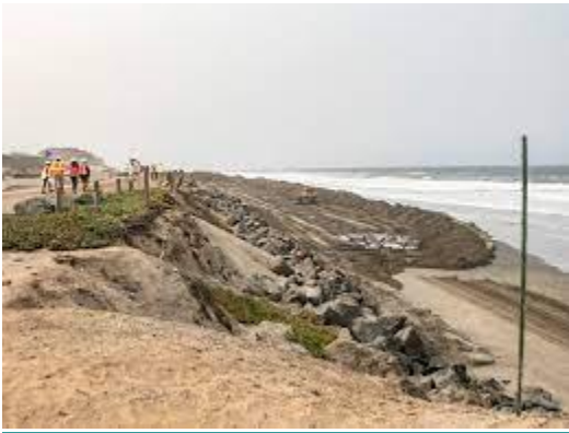
Sand being placed on Ocean Beach. Photo credit: U.S. Army Corps of Engineers
