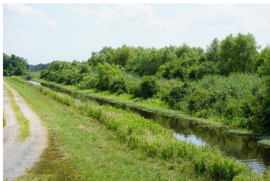
A drainage canal with a water control structure in Pocosin Lakes National Wildlife Refuge. Photo credit: NC Wetlands. Public domain.
