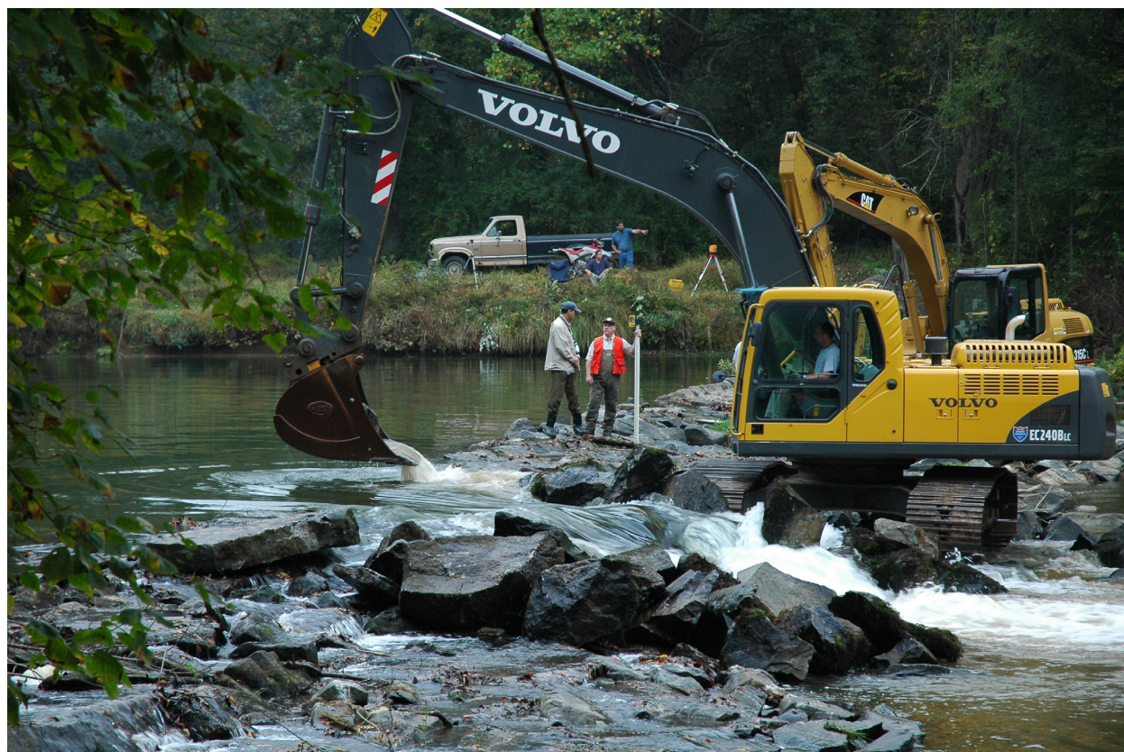
Figure 24.1 Dam removal on Octoraro Creek, MD
