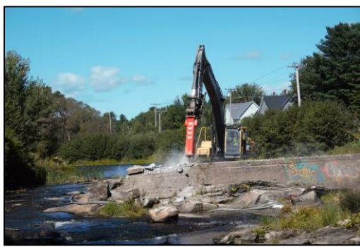
Construction crews demolishing a dam on the Sabattus River: Catherine Birmingham/ASF
