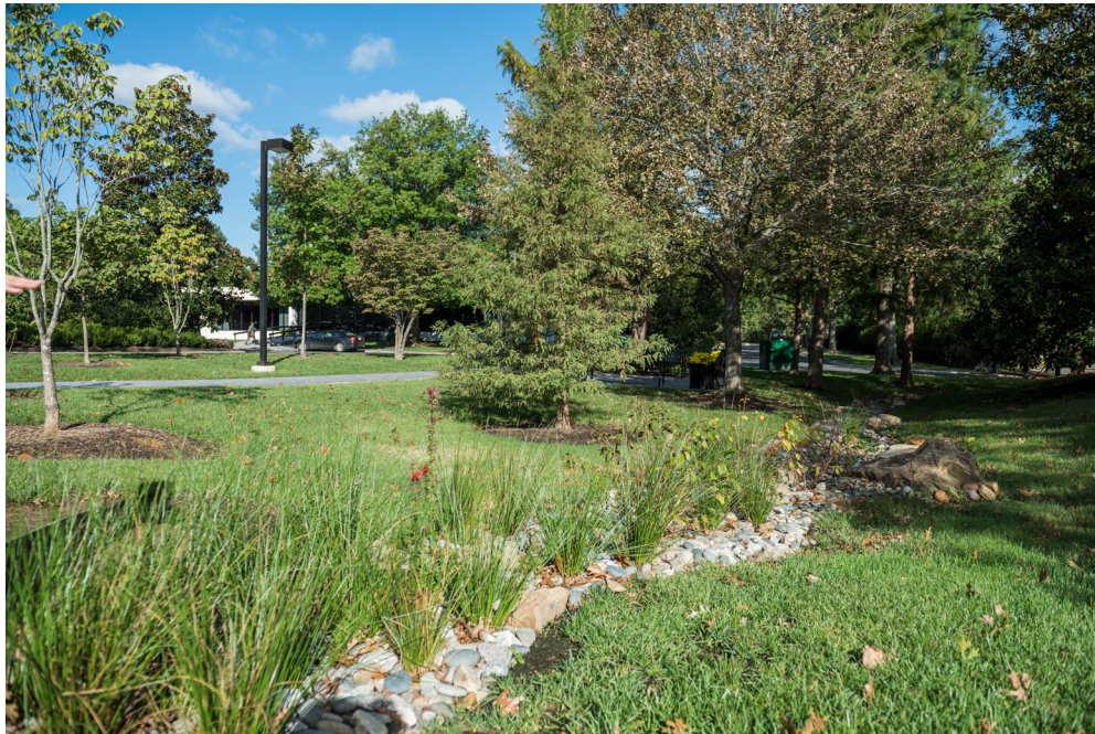
Figure 17.2 Bioswale at Arlington National Cemetery
