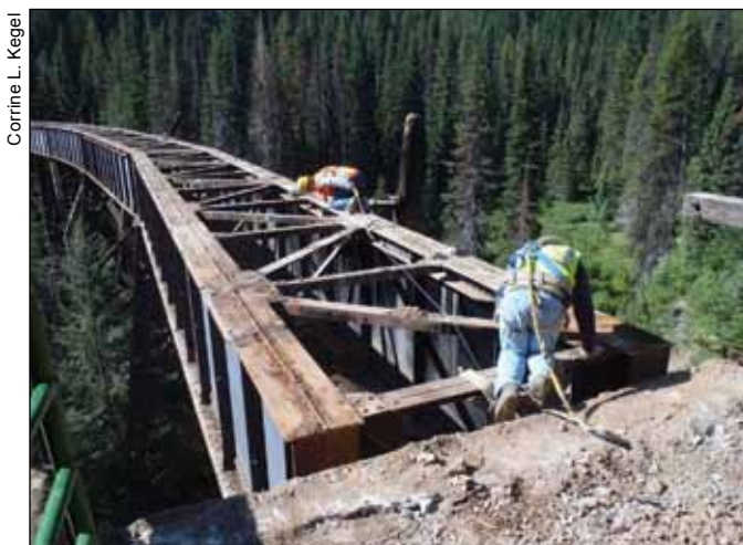
Figure 7-14—Dick Anderson Construction Company takes extra safety precautions while working on trestle repair.
