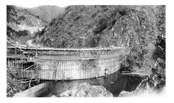
San Clemente Dam was constructed in 1912 on the Carmel River to provide water supply for the Monterey Peninsula. It was 106 feet tall and had a reservoir storage capacity of approximately 1,425 acre-feet.
