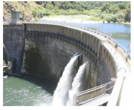
Once constructed, the reservoir quickly filled with sediment. Toward the end of its life, the reservoir was filled by more than 2.5 million cubic yards of sediment, leaving a storage capacity of only 70 acre-feet, or 5% of what it was built for. The dam no longer served a useful purpose.
