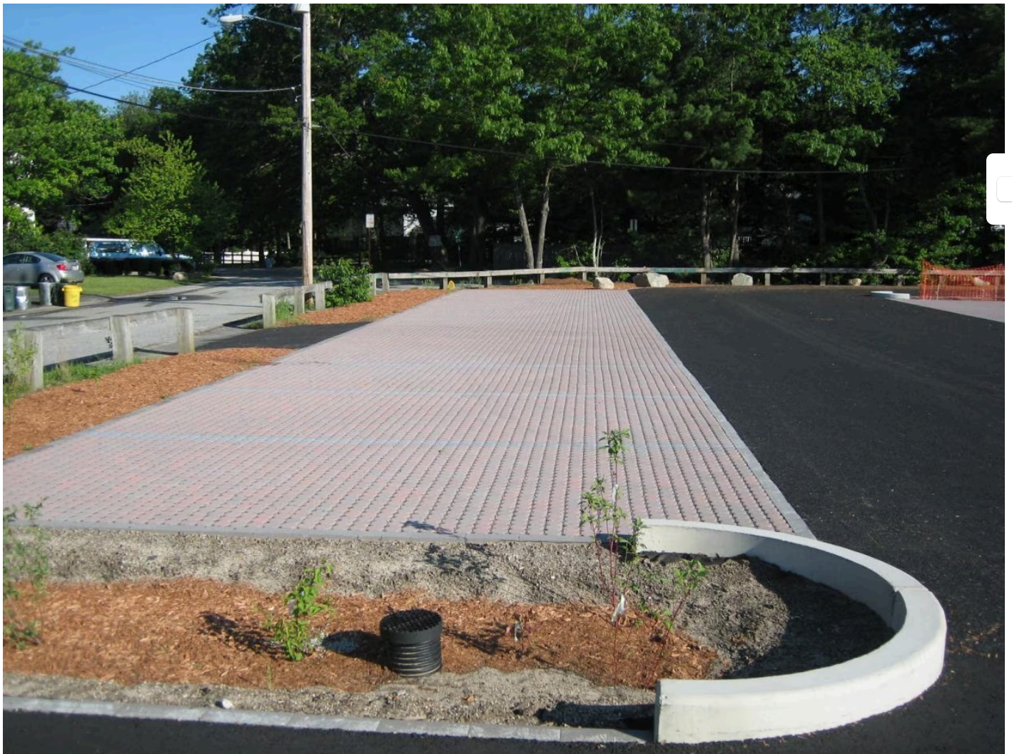
Permeable pavers, porous asphalt, and bioretention cells at the Silver Lake beach parking lot, Wilmington MA (photo: GeoSyntec)
