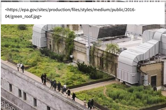
Chicago City Hall's Green Roof.
