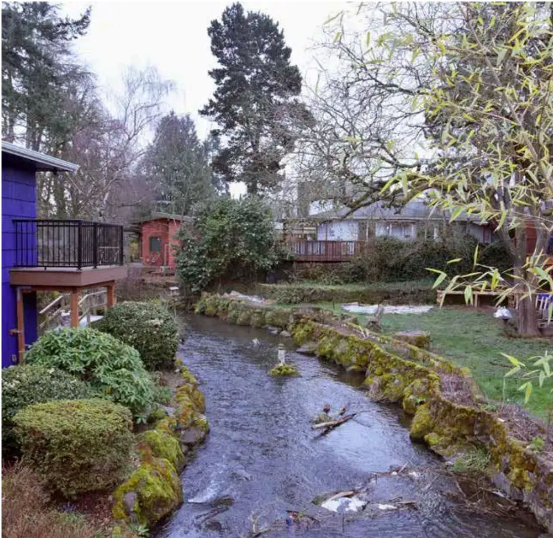
Woody debris, pools, and riffles in the restored Crystal Springs Creek just downstream of the Umatilla Street culvert.
