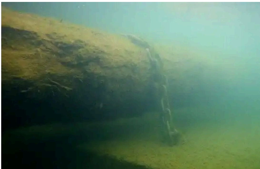
Anchors securing the woody debris to the river bottom.
