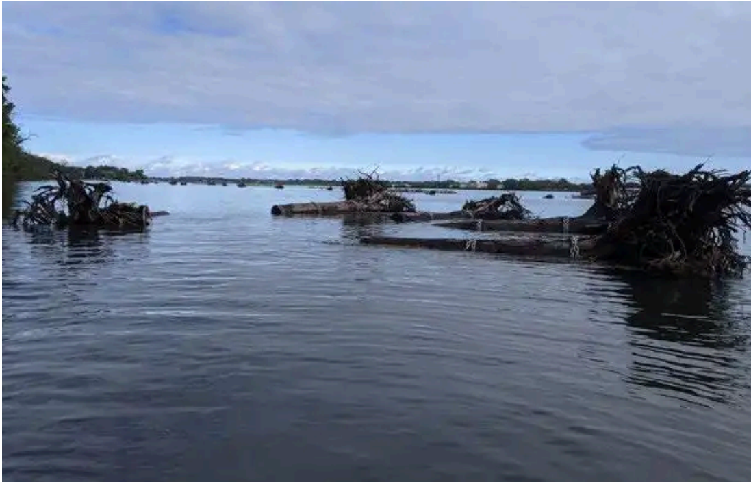
The ballasted woody debris provides wave attenuation and fish habitat. Construction of the wave-attenuating structures was completed using an excavator on a floating pontoon.
