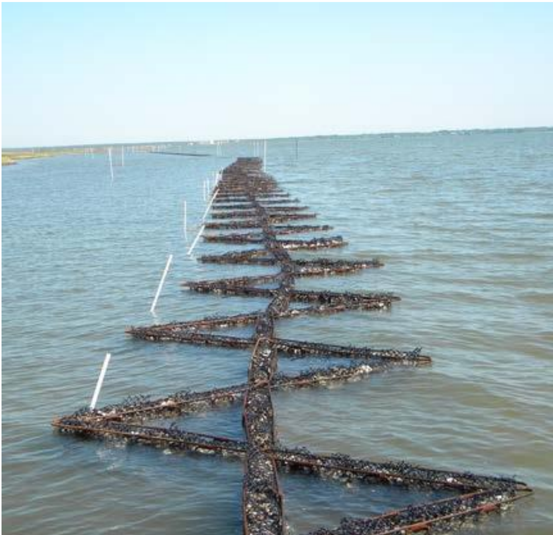
Oyster reef breakwater constructed from ReefBLK.
