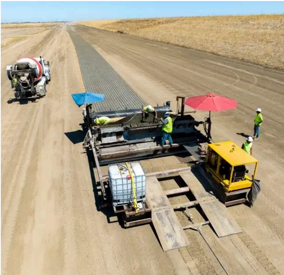
Fabrication of the tied concrete block mats before placement on the setback levee.
