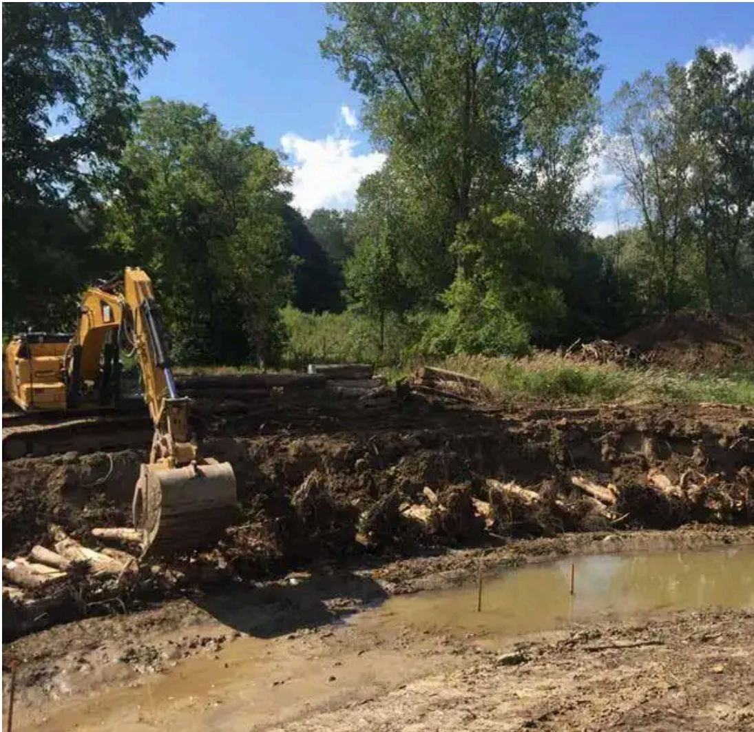
Installing root wads and stones to mimic natural features.
