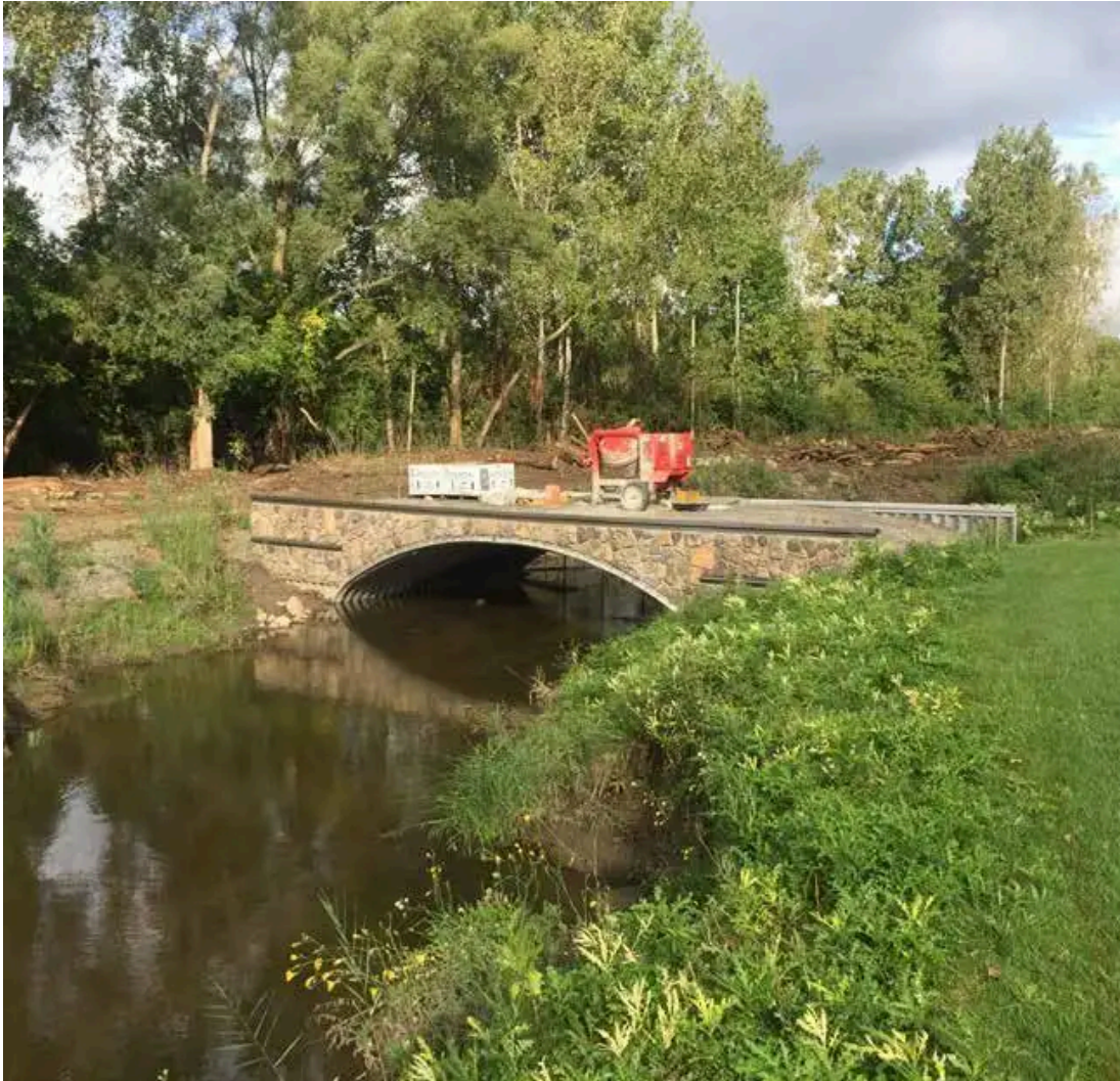
Increasing the size of the stream crossing for better fish passage.
