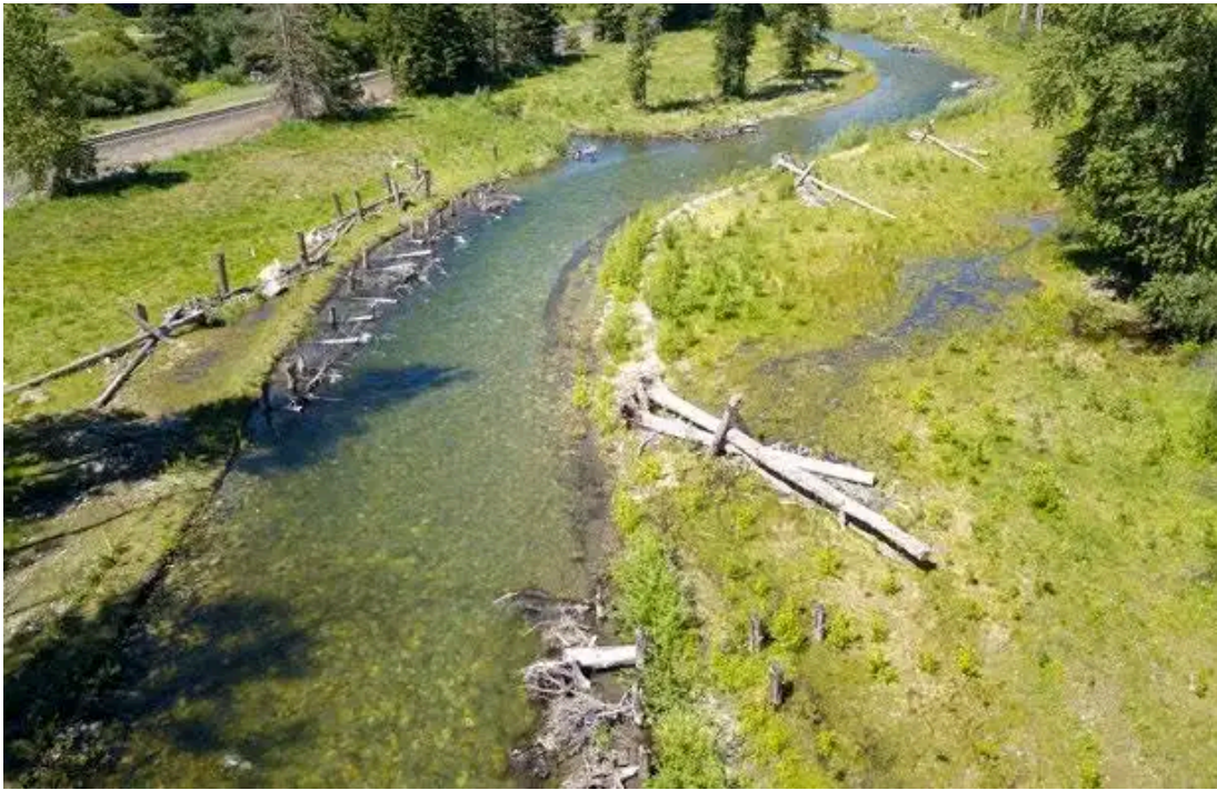
Aerial view of the site, taken three years after construction, showing the remeandered channel, large wood habitat, and vegetation growth on the new floodplain.
