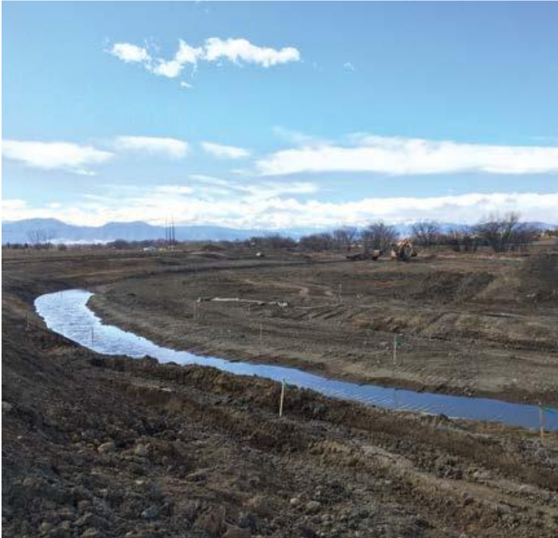
Lower Boulder Creek, channel meander and floodplain bench construction, 2016. (Photo by USACE Omaha District)
