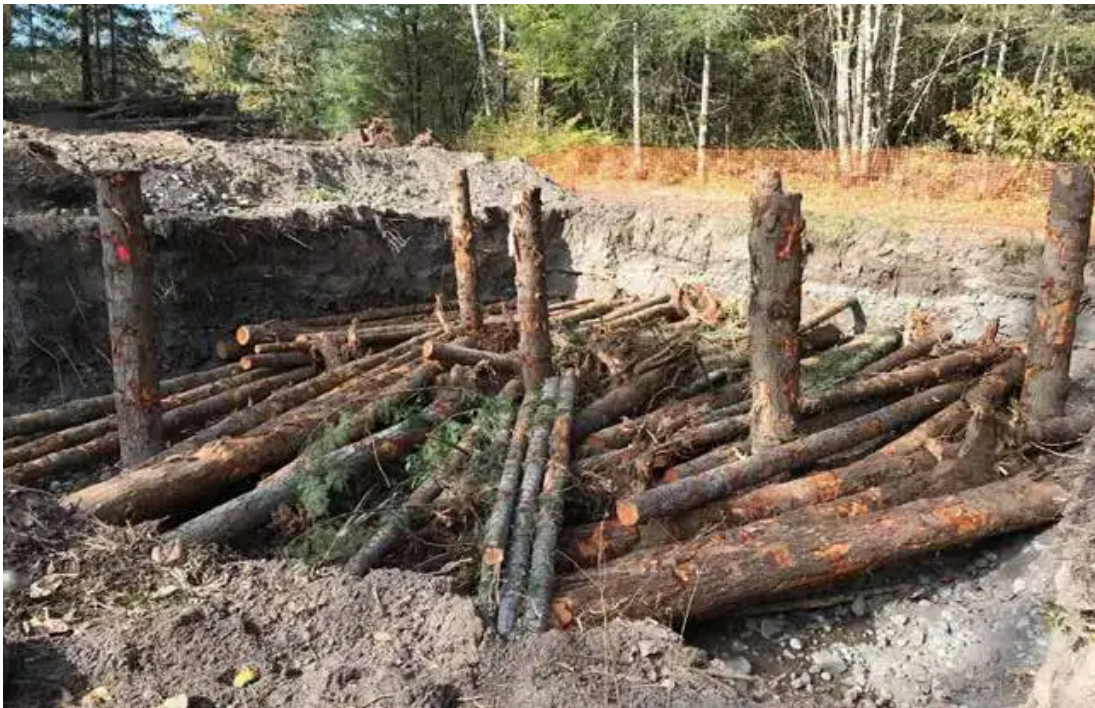
The base layer of the engineered log jam during construction.
