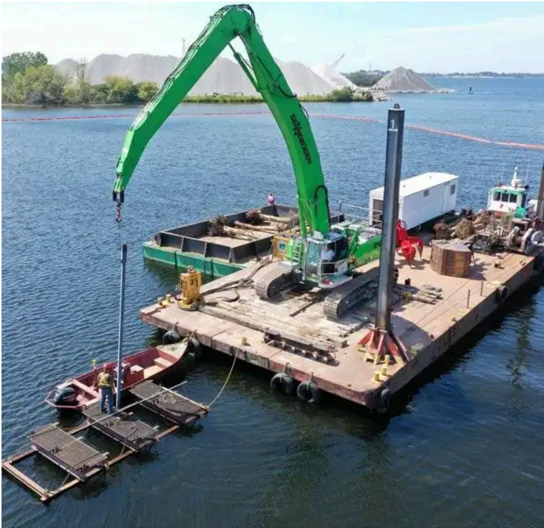
Shoal construction with an excavator on a floating pontoon.
