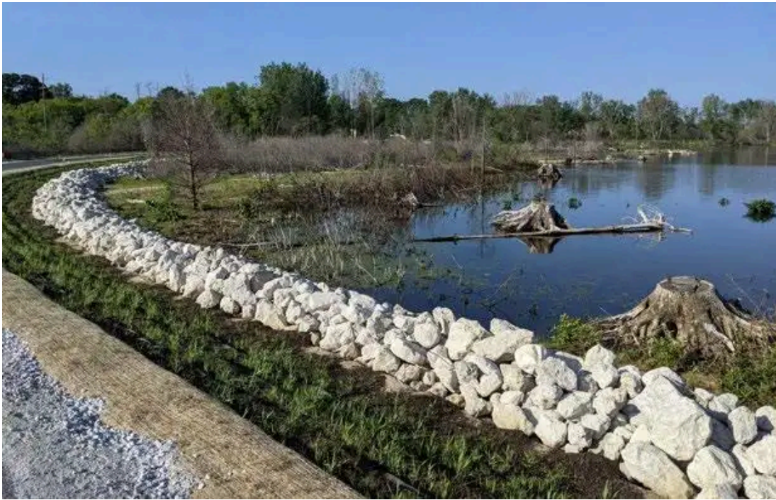
The wetland with compost and plantings over Envirolok with a riprap toe.
