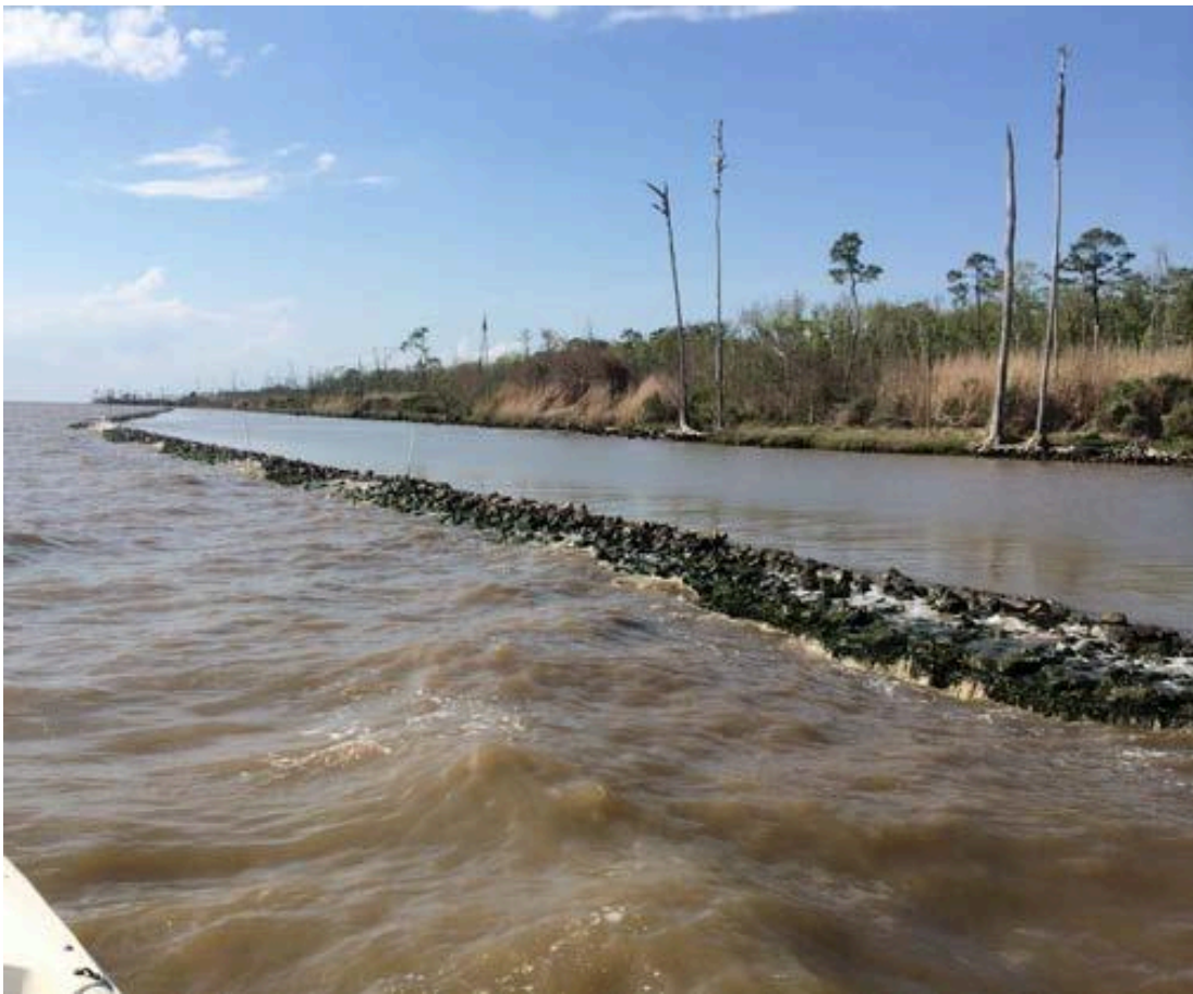
Breakwaters attenuating waves at Swift Tract.
