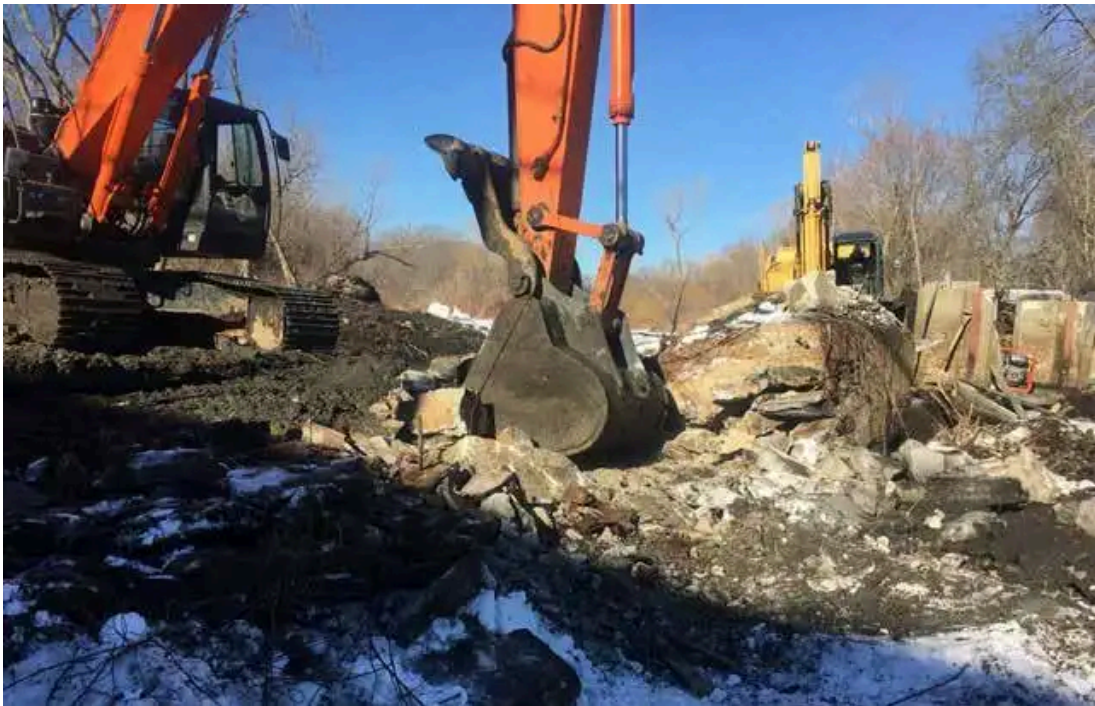
Demolition of the West Britannia Dam in 2018. (Photo by James Turek, NOAA Restoration Center)
