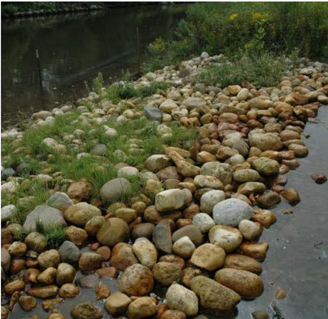
Cobble bars help prevent erosion and stabilize the banks.
