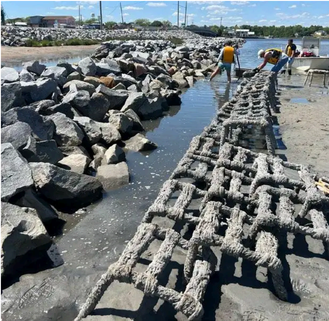
Installation of Oyster Catcher tables, a jute fiber and cementitious material matrix that has high oyster spat recruitment, thereby allowing for the creation of a new oyster reef.
