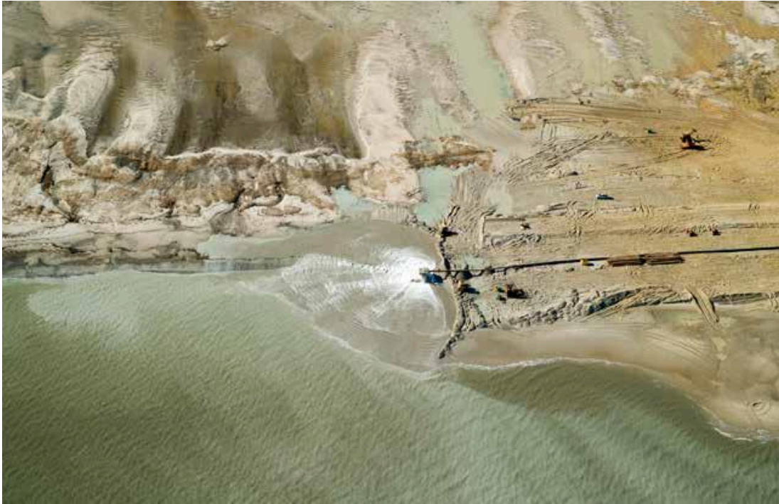
Bulldozers spreading sand after it is pumped onto the beach (Photo by TI Coastal Services Inc., courtesy of Norfolk Dredging Company)
