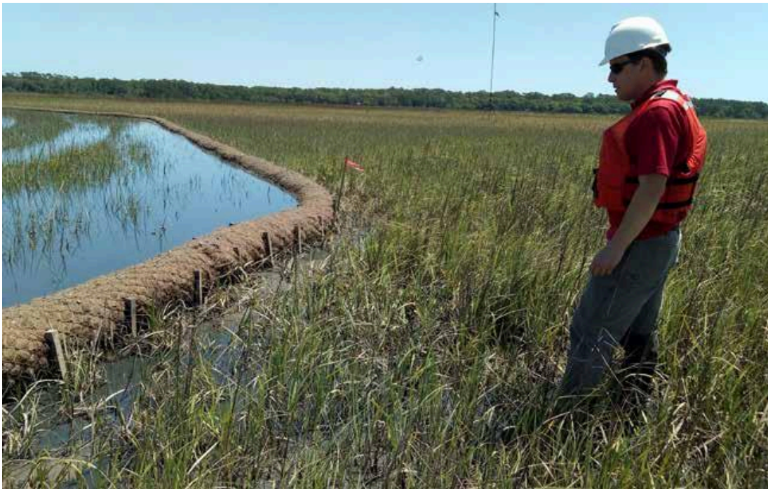
USACE project manager on site on the first day of sediment pumping. (Photo by Georgia Department of Natural Resources' Coastal Resources Division)
