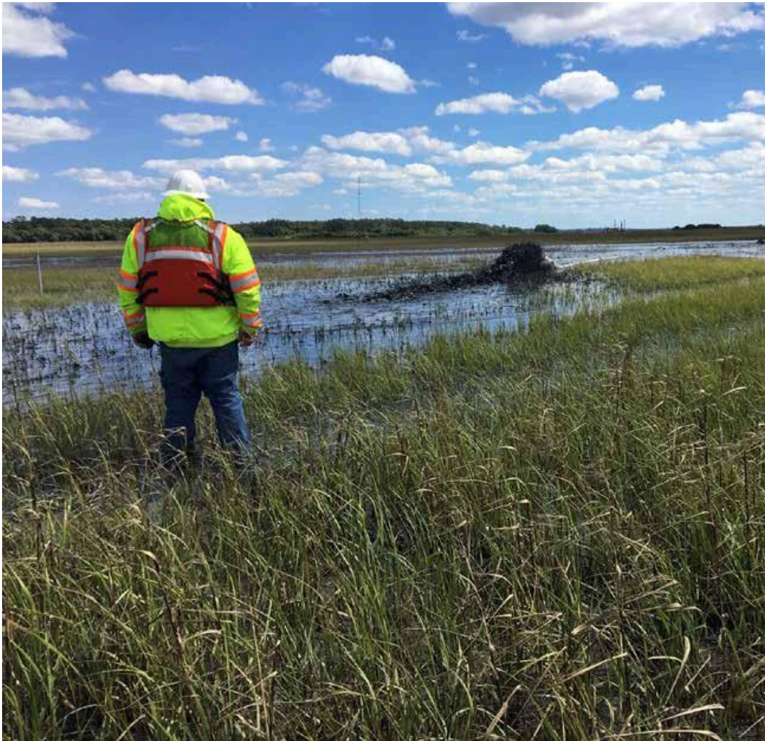
A dredging project manager monitoring dredged sediment placement in April 2019.
