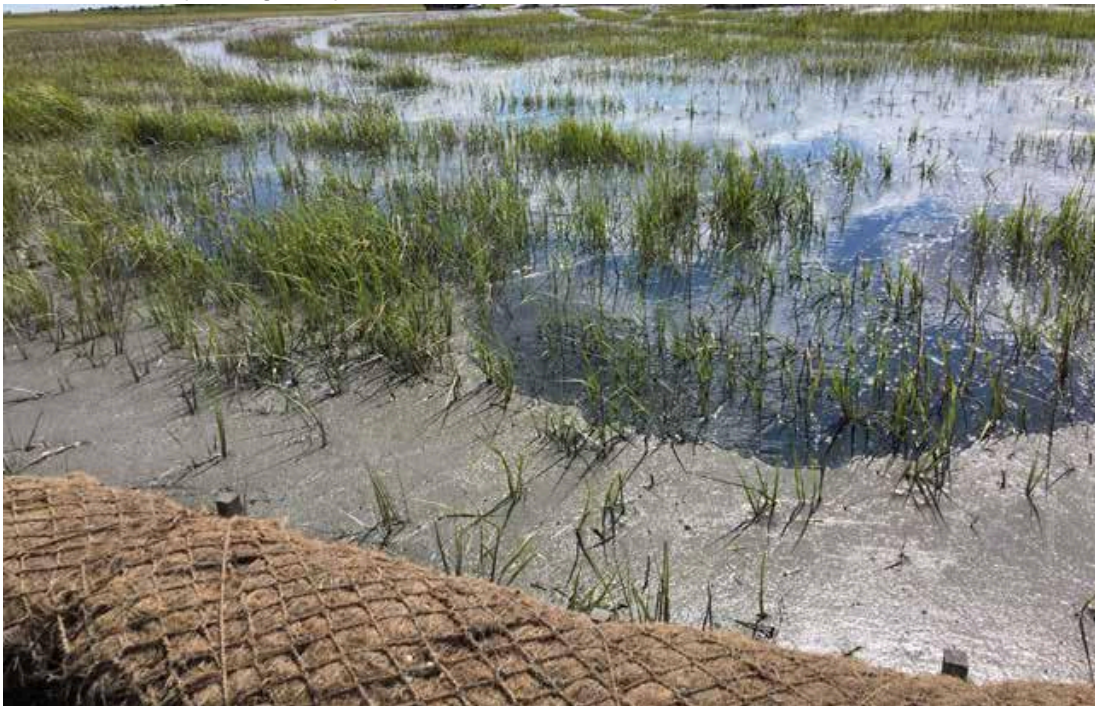
Dredged sediment spreading across the containment area. (Photo by Clay McCoy, USACE Jacksonville District)
