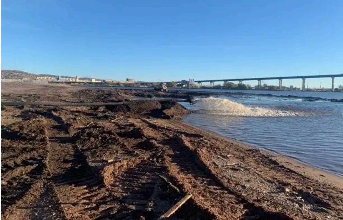
Active hydraulic placement of dredged material at Interstate Island. A baffle plate is attached at the end of the pipe at a 45-degree angle to dissipate the energy from the flow of the dredged material out of the pipe to help minimize turbidity.
