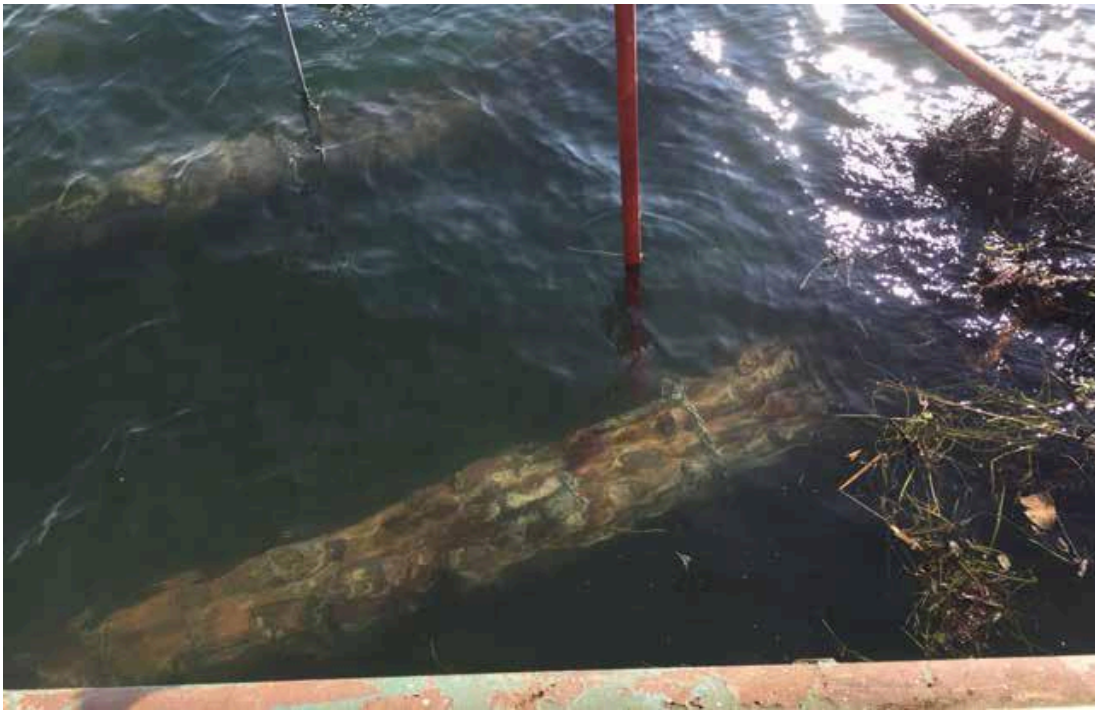
Earth anchors securing the root wads to the lake bottom. (Photo by Keith Kropfreiter, USACE Detroit District)
