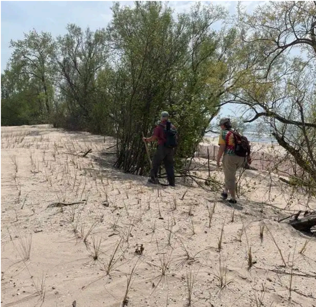
The newly constructed dune with dredged sand and rows of transplanted beach grass. This dune has continued to accrete with sand from aeolian drift captured by the beach grass.
