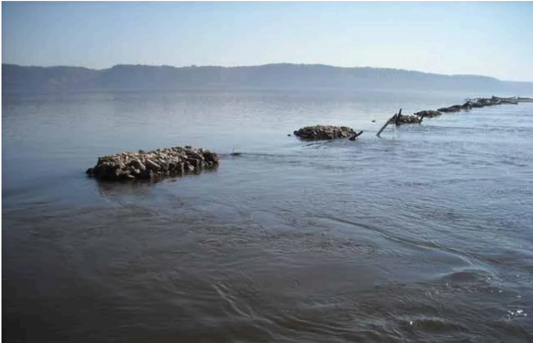
A rock and log sill installed in the river to increase the flow in the area during flood events. (Photo by USACE St. Paul District, Eastern Area Office)
