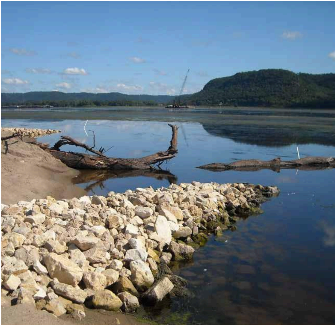
A rock vane and loafing structure integrated into a newly constructed island in 2011.
