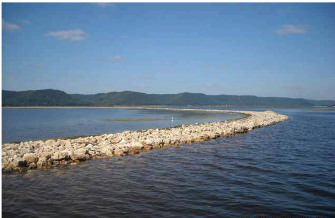
A rock sill redirects water during high-flow events. (Photo by USACE St. Paul District, Eastern Area Office)
