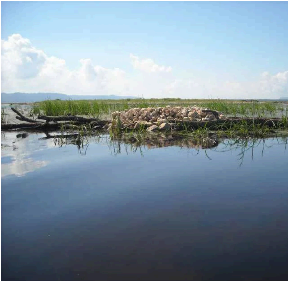
A well-established seed island has formed due to sediment accumulation in the deposition zone behind a wildlife loafing structure, or large woody debris, in 2010.
