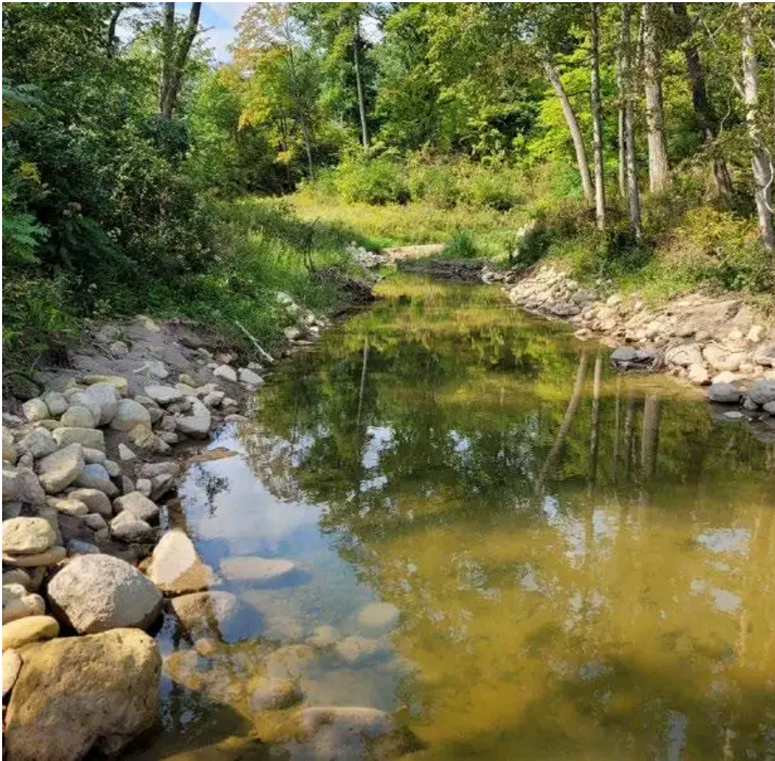
Restored ravine stream with rounded cobble for erosion protection. (Photo by USACE Chicago District)
