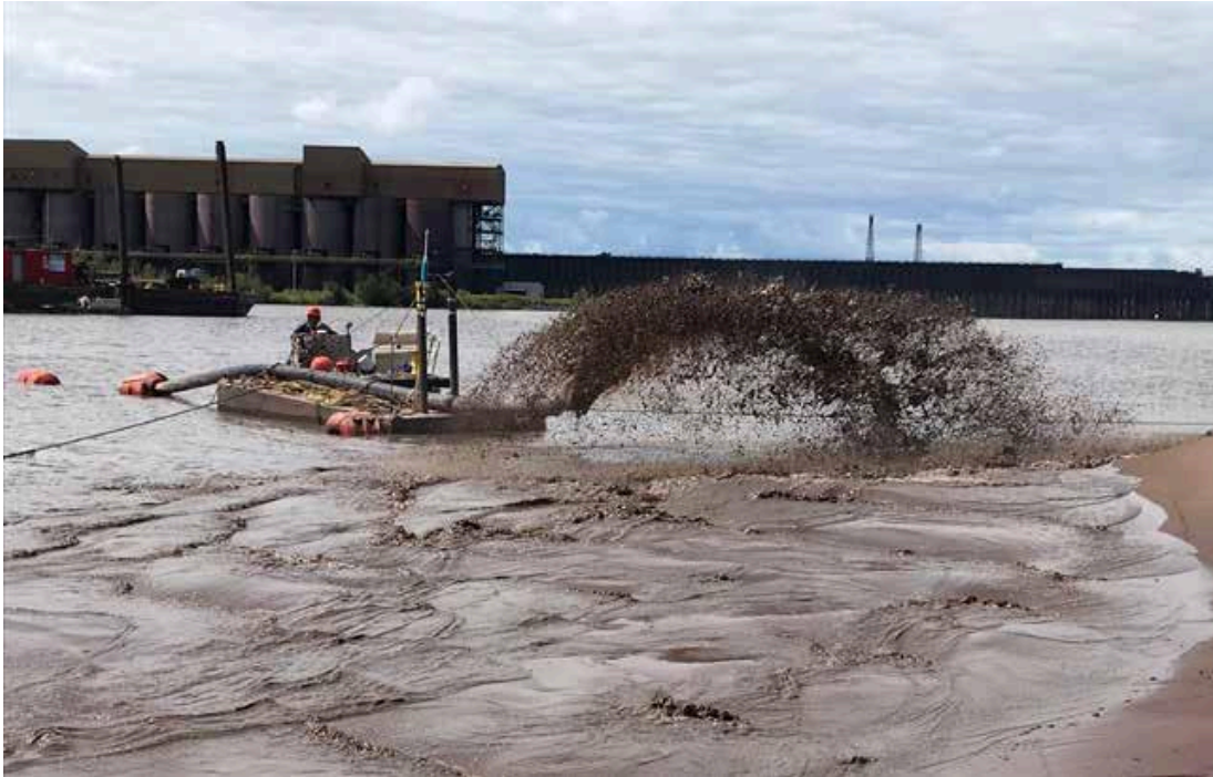
Dredged sediment was hydraulically placed to create piping plover habitat.
