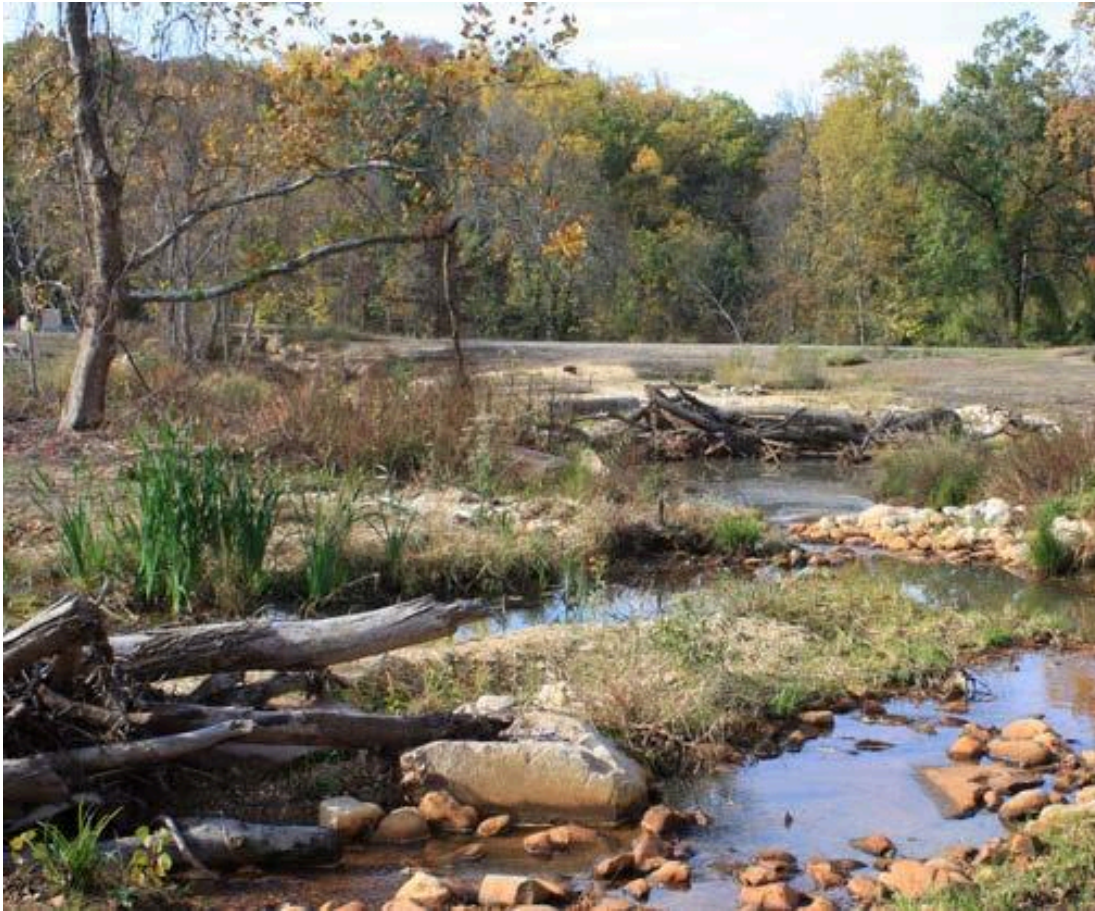
Adding natural pools and riffles improved diversity and quality of in-stream habitats. (Photo by Tim Welp, ERDC)
