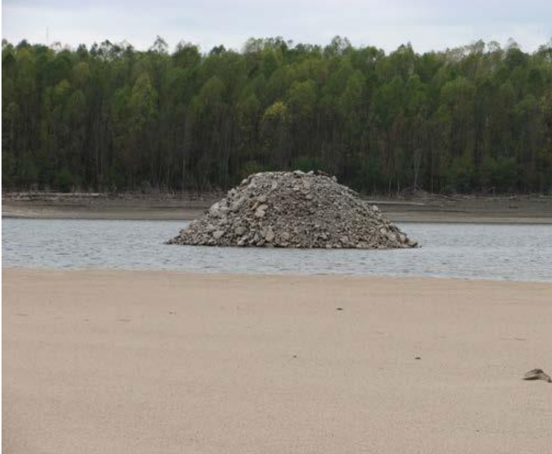
This photograph shows a stone roundpoint structure creating habitat complexity within the secondary channel.
