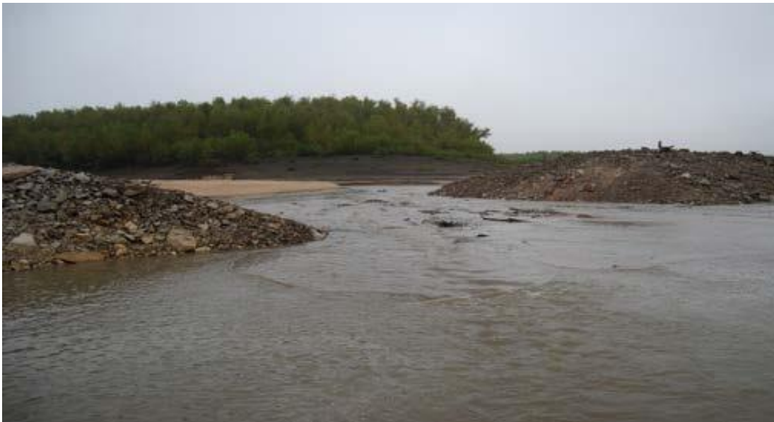
Flow during low-water stages is restored through a notched dike within the secondary channel.
