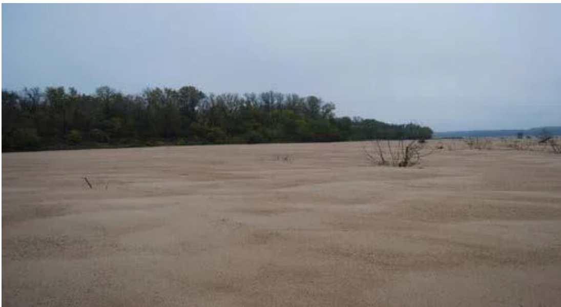
This photograph shows sand deposition within the secondary channel during low-water stages prior to restoration efforts.
