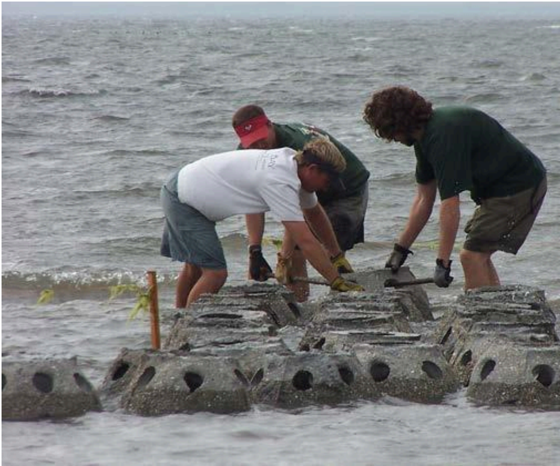
Volunteers place Lo-Pro Reef Ball units (or concrete oyster domes) by hand to facilitate the creation of oyster reef in the intertidal environment.
