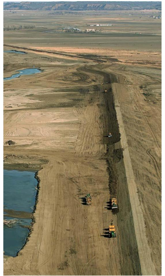
Work in 2012 repairing the middle breach in levee L-575 near Hamburg, lowa, is substantially complete. The setback levee restores the level of risk reduction at the site to its preflood status.
