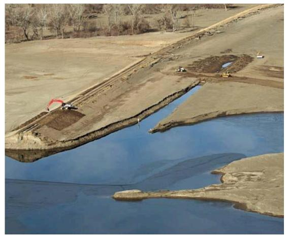
Work repairing the lower breach in levee L-575 began recently with construction crews placing hydraulic fill into scours and beginning to build the base for the setback levee alignment. The work will restore the level of risk reduction at the site to its preflood status. (Photo by Kevin Wingert, Systems Restoration Team, USACE Omaha District)
