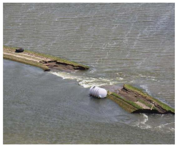
An aerial view of an intentional breach in levee L-575 near Hamburg, Iowa, 2011. The intentional breach was created by the local sponsor and approved by USACE following a full breach of the levee. The intentional breach was conducted by the sponsor to delay the time in which the area behind the levee would flood. The levee is located at River Mile 552 in Atchison County, MO.
