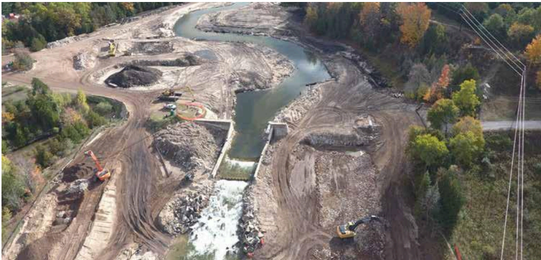
Sabin Dam and pond in the last stages of drawdown, following demolition of a majority of the powerhouse. (Photo by Brett Fessell, GTB Natural Resources)
