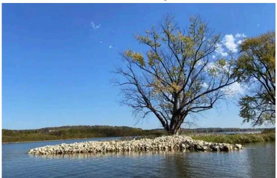
Rock was placed on the head (north end) of the island to create a bullnose to deflect the river's energy and limit flow erosion.
