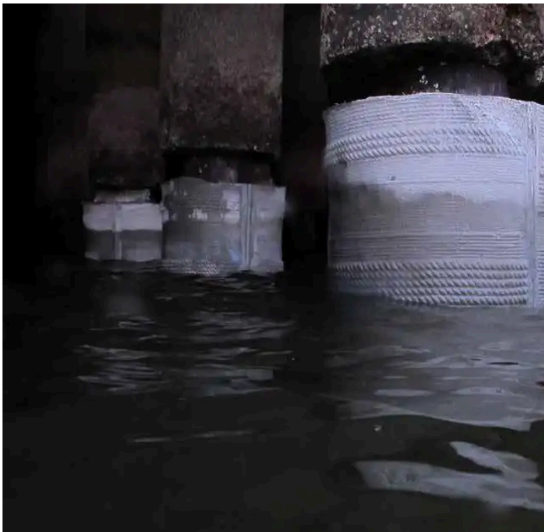
Pile encasements at time of installation in 2013 prior to the growth of marine organisms. (Photo by EConcrete Inc.)
