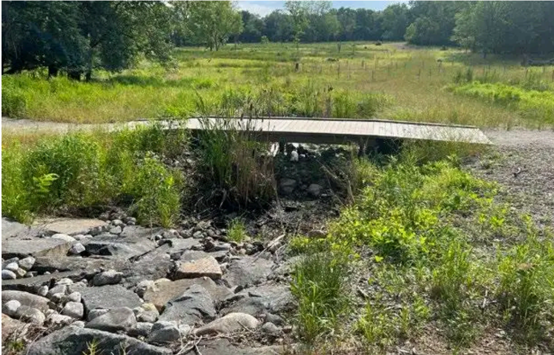
Regenerative stormwater conveyance (RSC) discharge under a boardwalk to the sand seepage network. A similar sand seepage wetland design approach was undertaken in an agricultural watershed at Bishopville, Maryland, in 2011.
