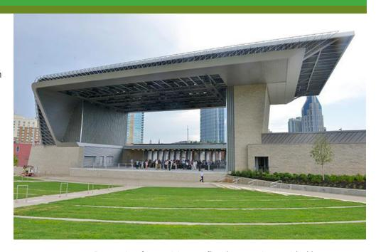
Protection from 500-year flood events is provided by an integrated flood wall that was built two feet above the 2010 flood levels. The wall doubles as seating and is not instantly recognizable as a flood protection feature, in keeping with the "park first" mandate for all features of the development.
