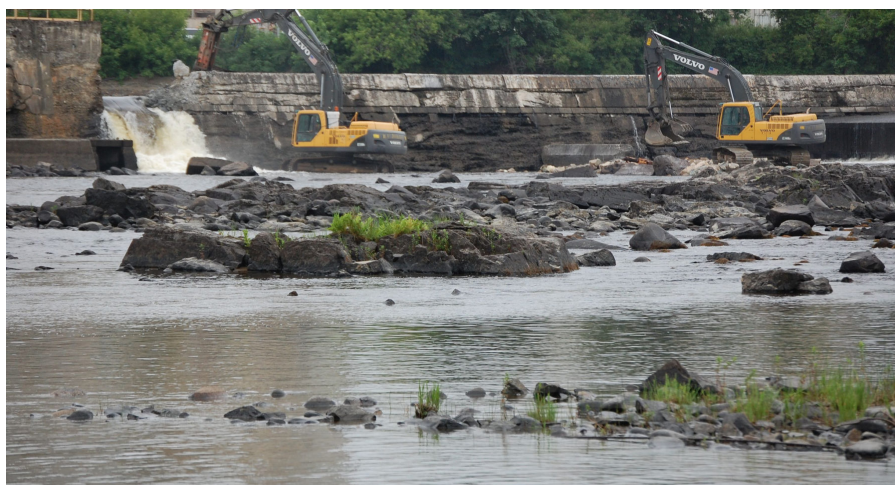
Breaching the Great Works dam where construction began in June 2012 which would be the first of two major dam removals. Obtained from Penobscot River Restoration Trust online files. – https://www.flickr.com/photos/penobscotrivertrust/7431203902/in/album-72157630262350632/
