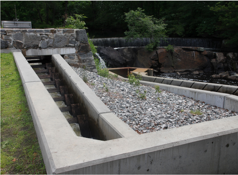
Credit: Brian Murphy, U.S. Army Corps of Engineers. Fish ladder at Hunt's Mill Dam.
