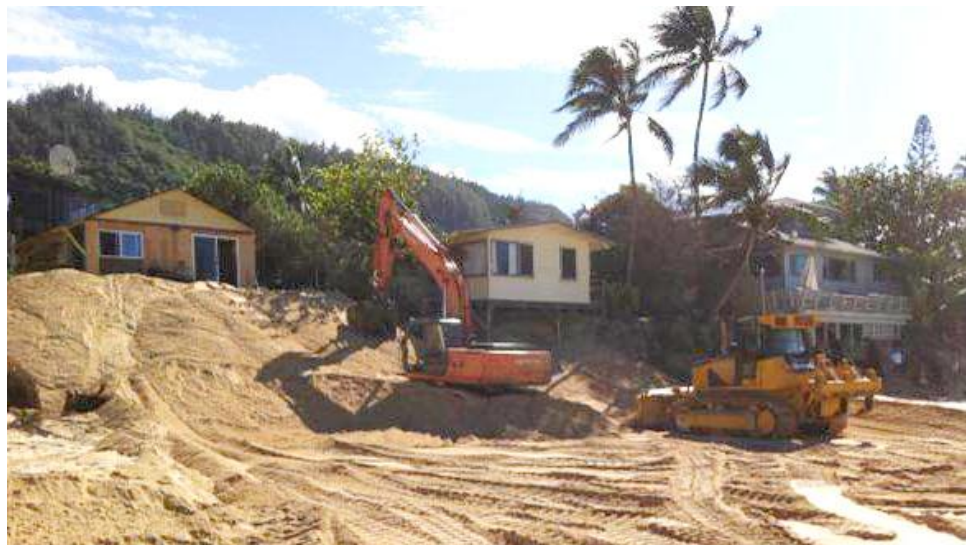
Construction equipment is used to restore dunes on the North Shore of O'ahu. This is one example of “soft” alternatives to hard armoring that can preserve the natural character of beaches while protecting homes from damage during high wave and storm events.
