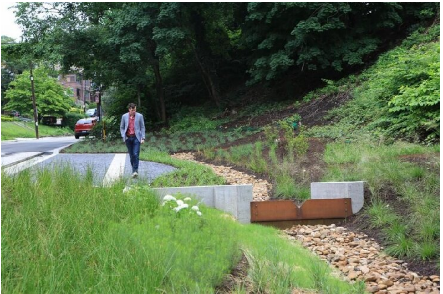
A section of the Centre and Herron stormwater project.
