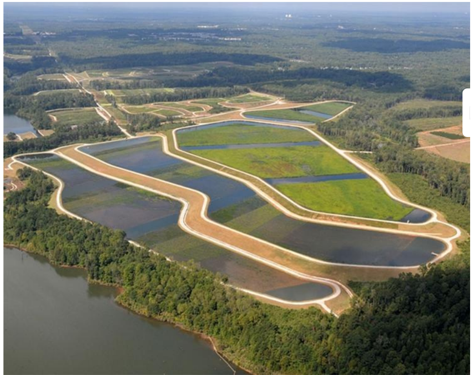
The E.L. Huie Jr. Constructed Treatment Wetlands is one of 28 major capital improvement projects that was completed as part of CCWA's Water Resources Initiative 2000 Master Plan. These wetlands provide a sustainable system for Clayton County.
