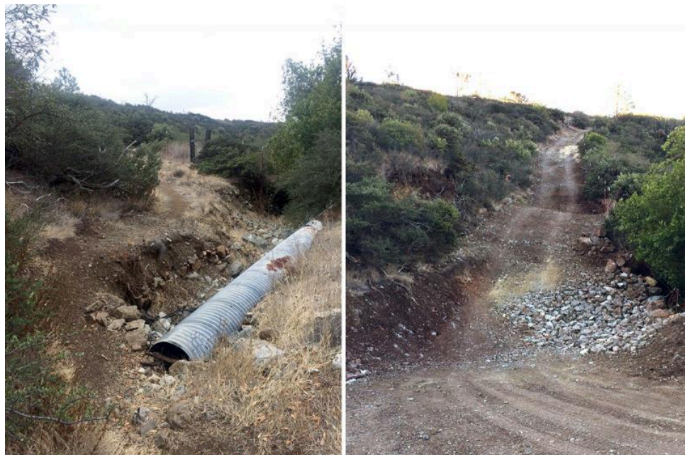
Before (left) and after (right) photos show the results of a project to reduce sedimentation from roads in Morro Bay's upper watershed. Before the project, streams eroded around this culvert and carried soil from a loose-surface road into the bay. The culvert was removed and the road was upgraded with armored fill.
