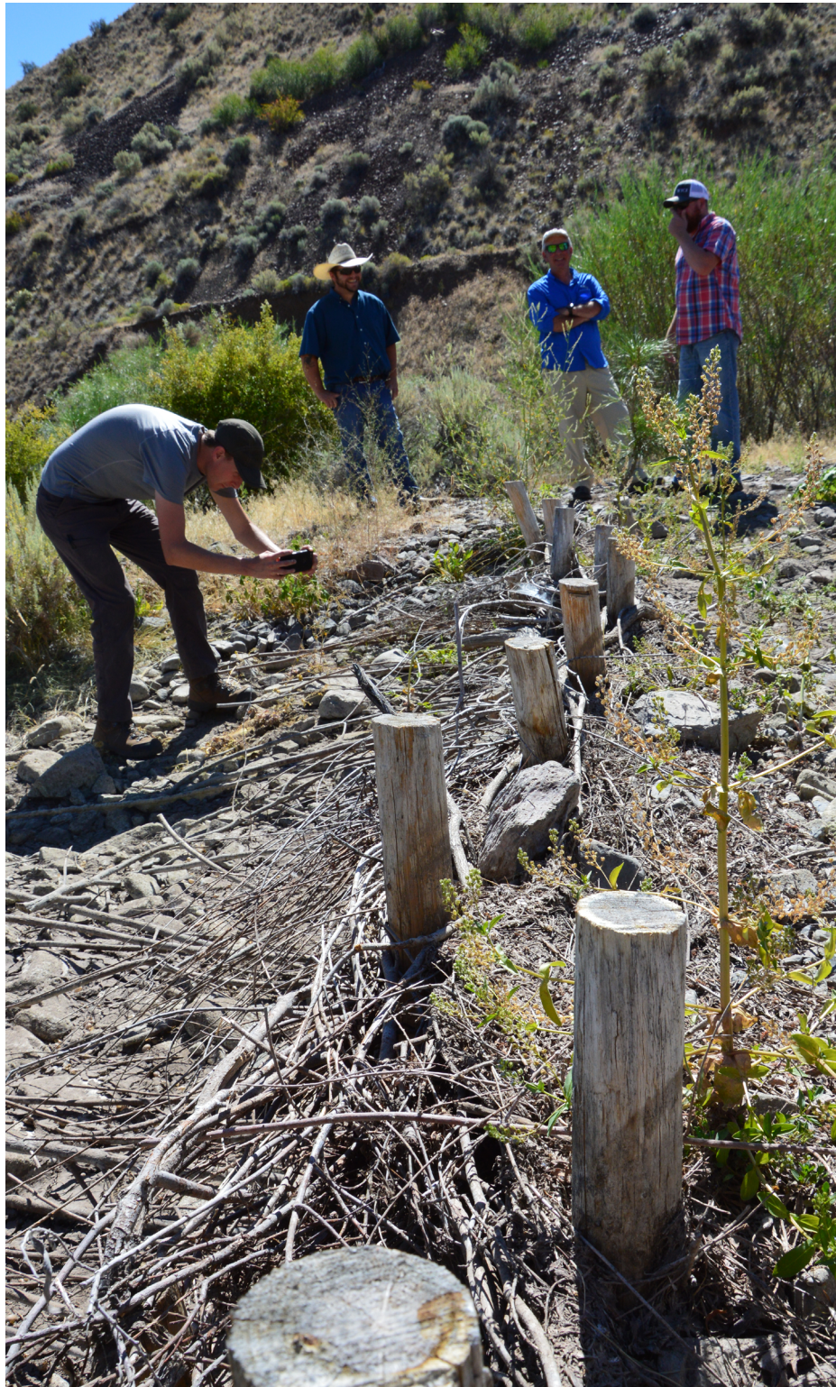
Figure 21.1 Beaver dam analog at the North Slope Ochoco Holistic Restoration Project, OR
