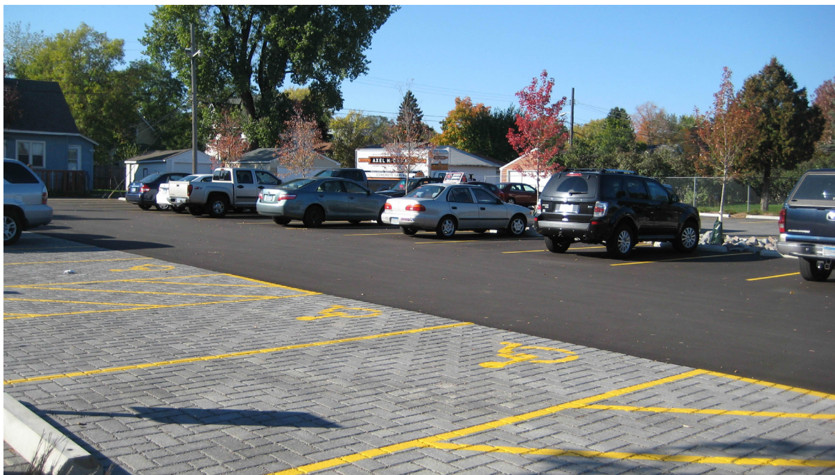
Figure 17.4 Permeable pavement in a Mississippi high school parking lot
