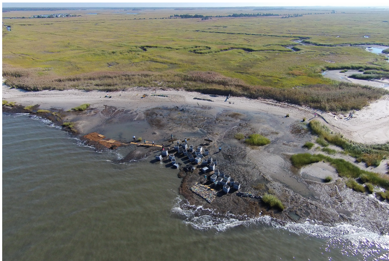
Figure 6.2 Aerial view of living shoreline construction using oyster castles
