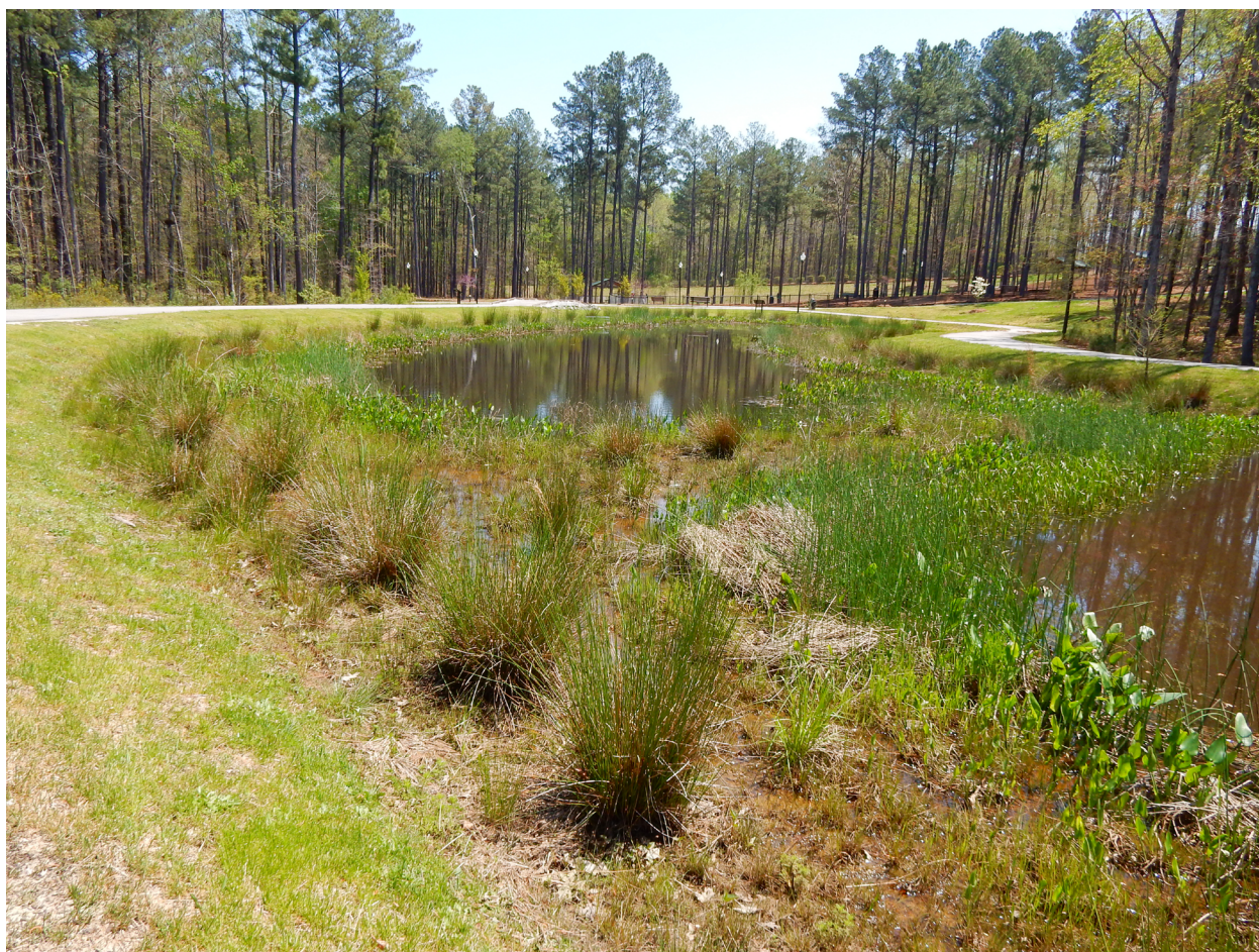
Figure 15.1 A stormwater treatment wetland in Apex, NC
