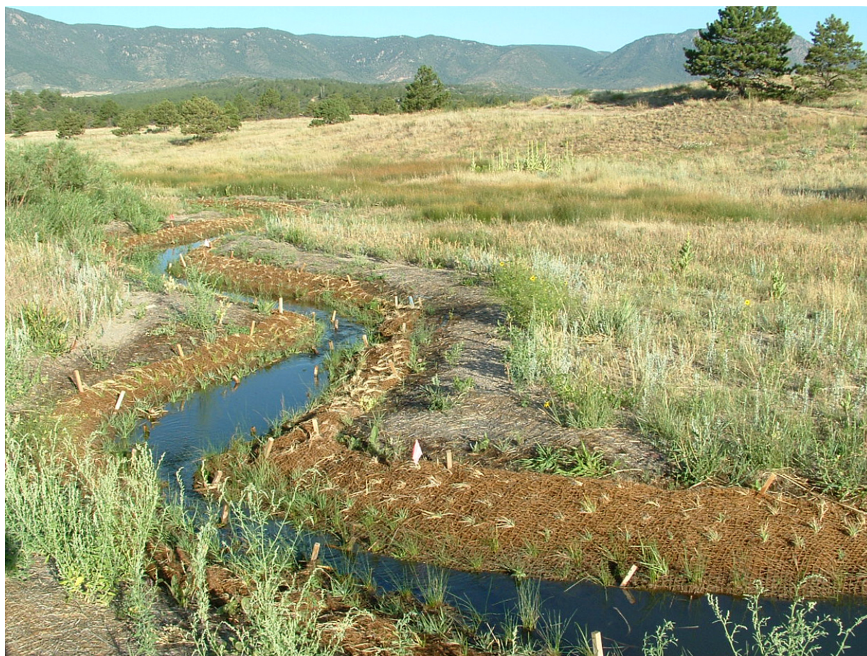
Figure 22.2 Constructed channel with reconnected floodplain at Black Forest Creek, CO
