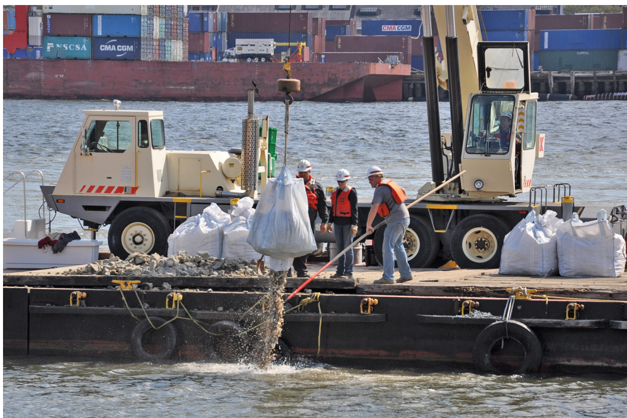
Figure 8.1 Depositing shell material into the water to create an oyster reef
