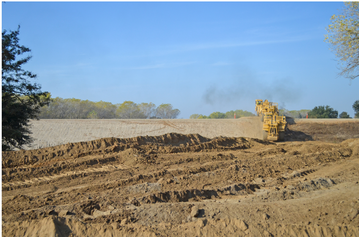
Figure 22.1 Construction equipment traverses a new setback levee to remove material from the old levee along the Sacramento River
