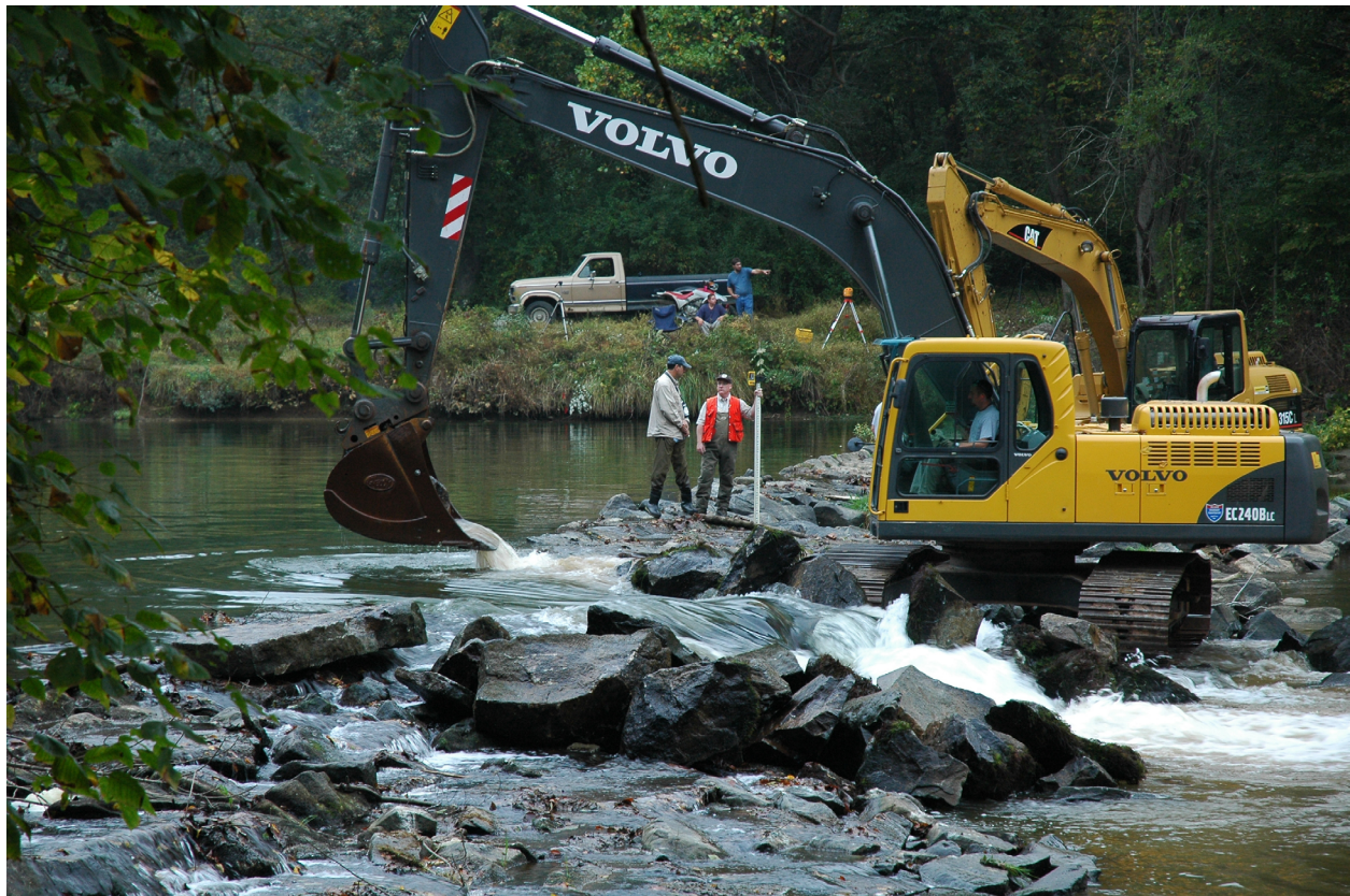
Figure 24.1 Dam removal on Octoraro Creek, MD
