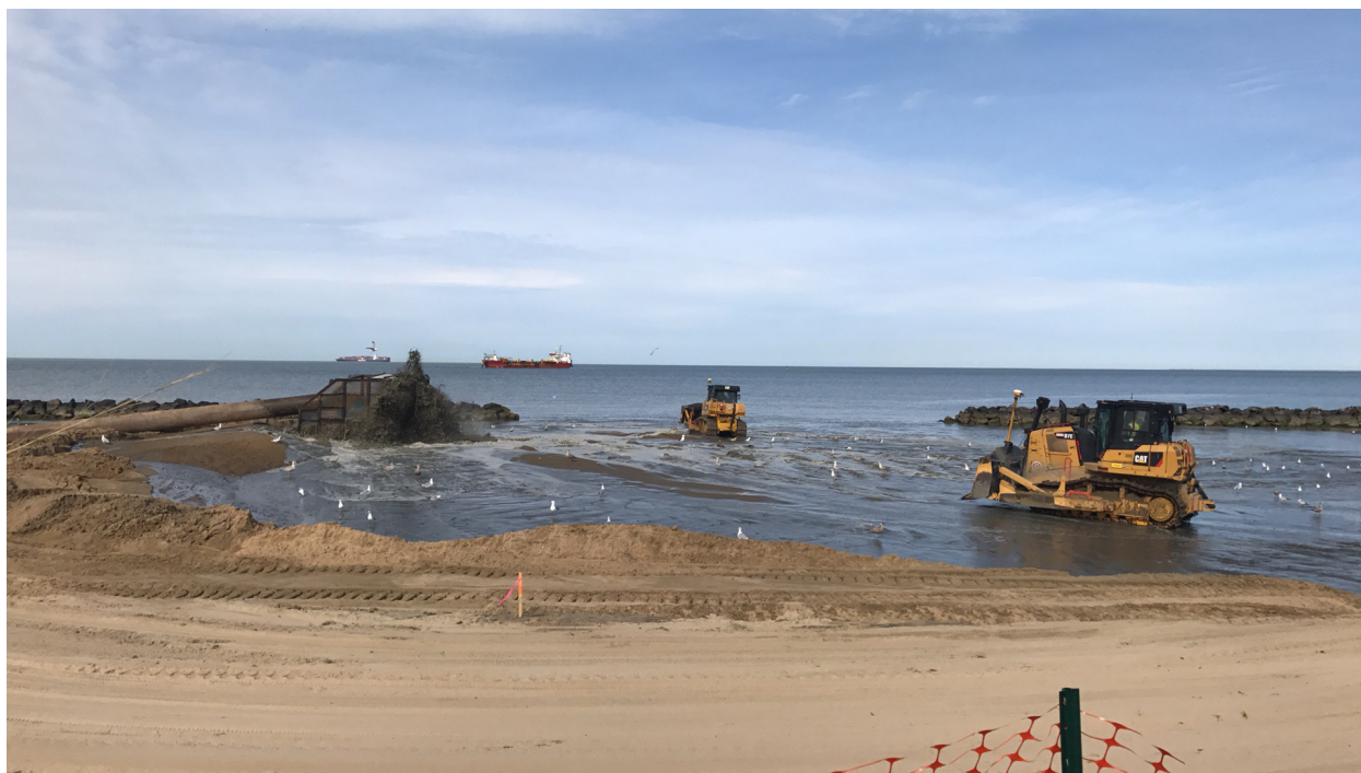
Figure 2.1 Nourishment of Ocean View Beach in Virginia via dredging and sand redistribution
